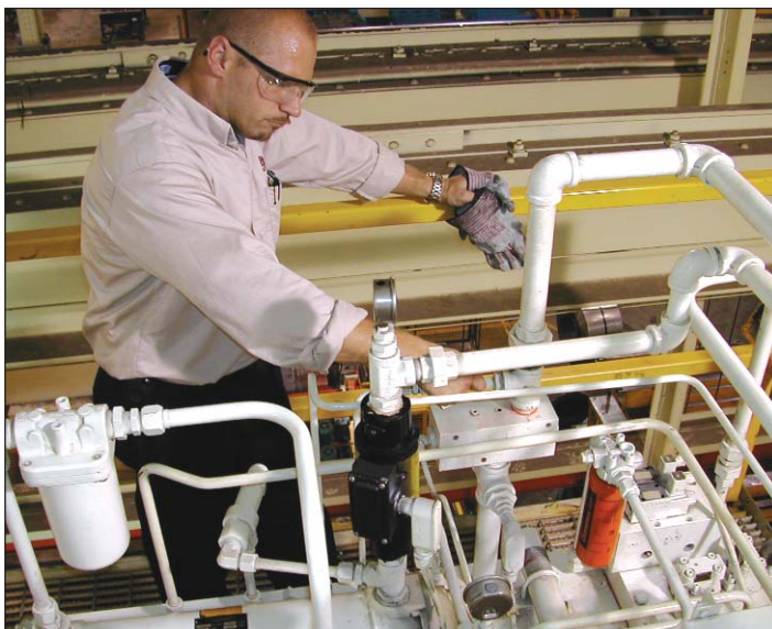
Hydraulic and Pneumatic Systems Inspection
