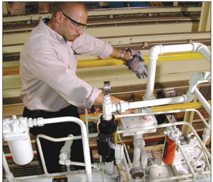
Hydraulic and Pneumatic Systems Inspection
